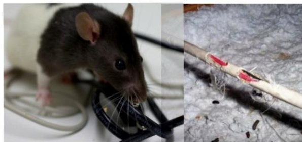
Rodent Chewing Cables
